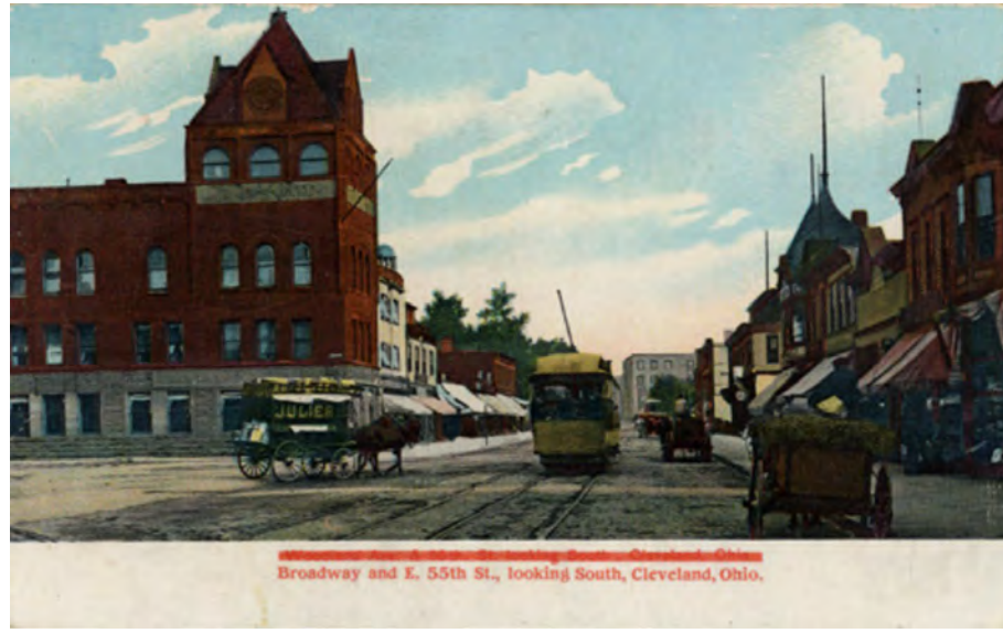
Litho-Chrome Postcard, c. 1900-1925 Broadway and E. 55th St., looking South (Project site not shown, Kresge Bldg. constructed in 1925)
